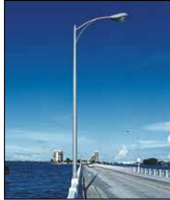
Venetian Causeway Miami, FL Installed Circa 1951
